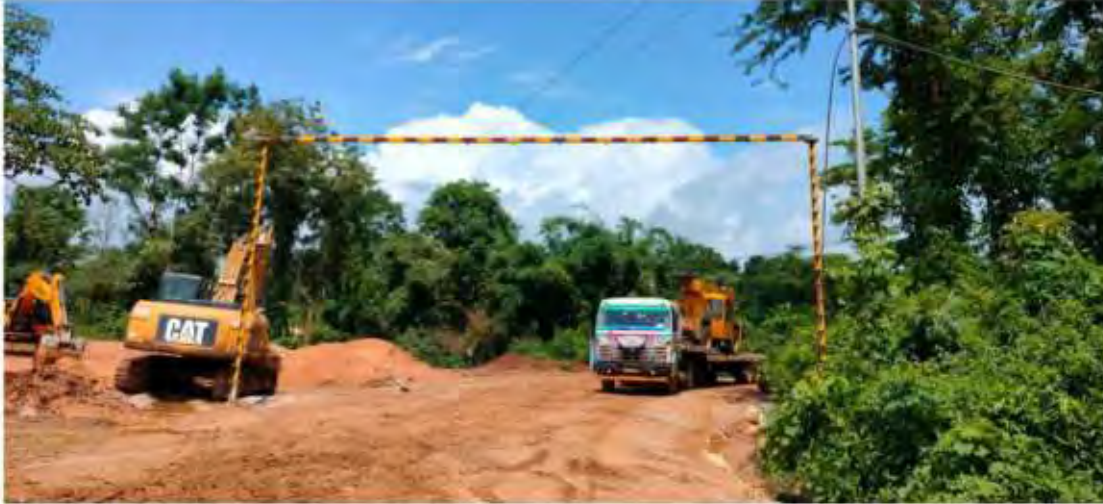
Fig -15. Goal post for overhead electrical line
