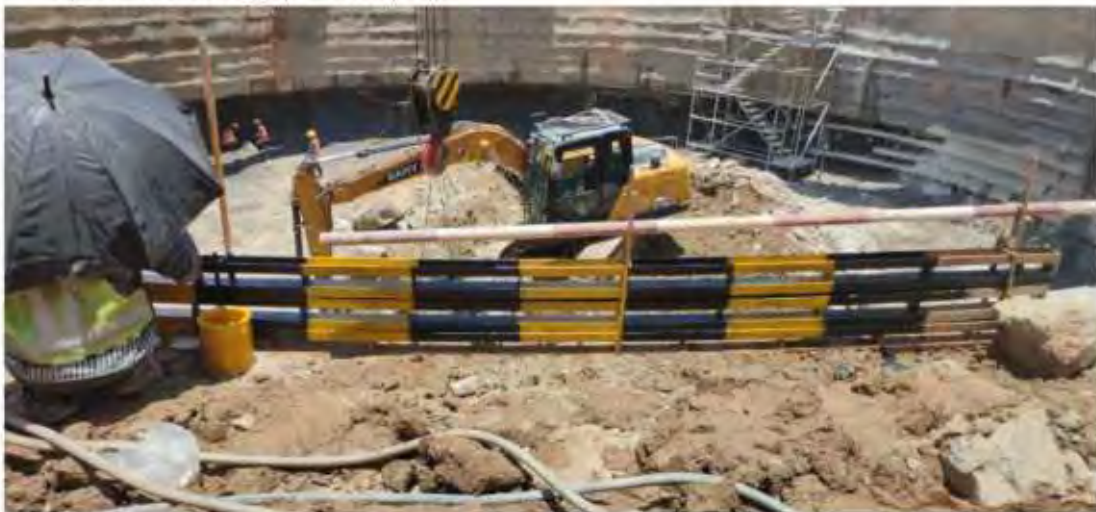
Fig -14. Hard edge protection for Surge Shaft deep excavation
