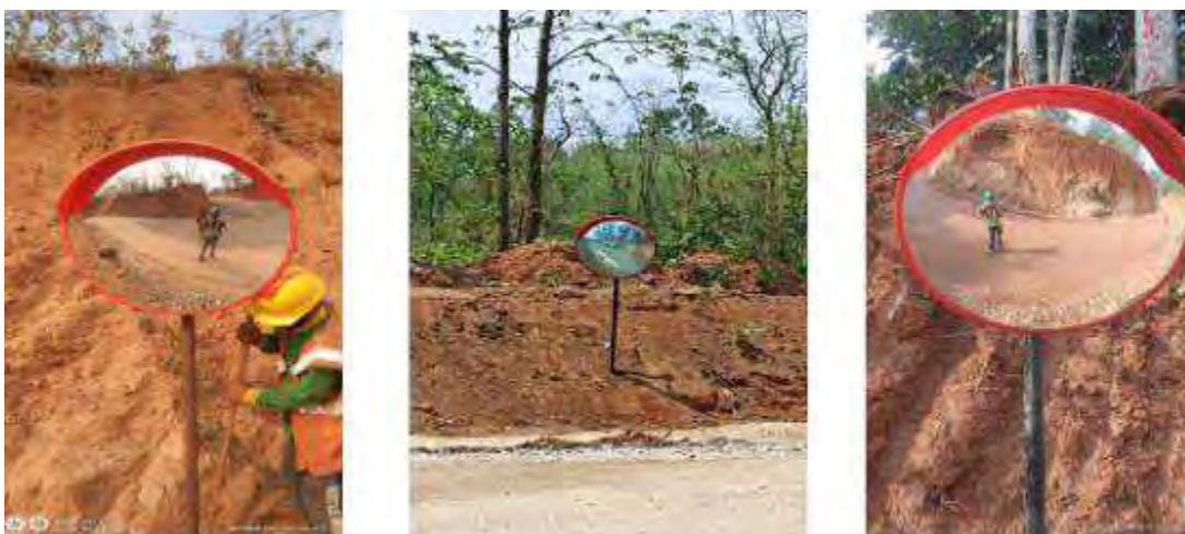
Convex mirror installed for blind corner of the site road
