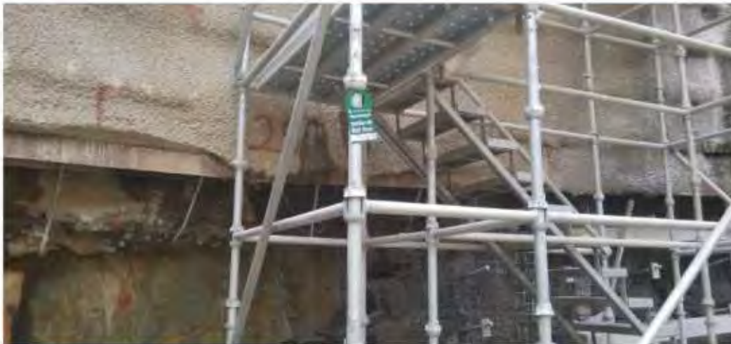
Fig -10. Scaffolding inspection Green Tag implemented
