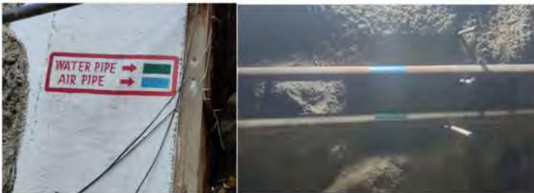
Fig -12. Color Coding for Tunnel air / Water pipeline.
